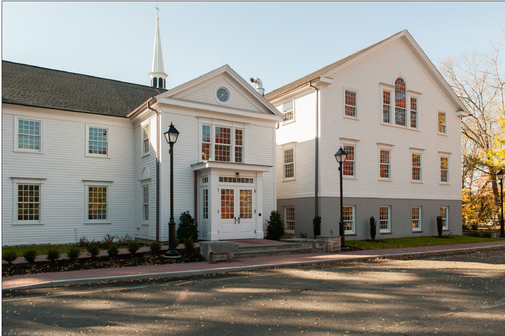
View from the Parking Lot
